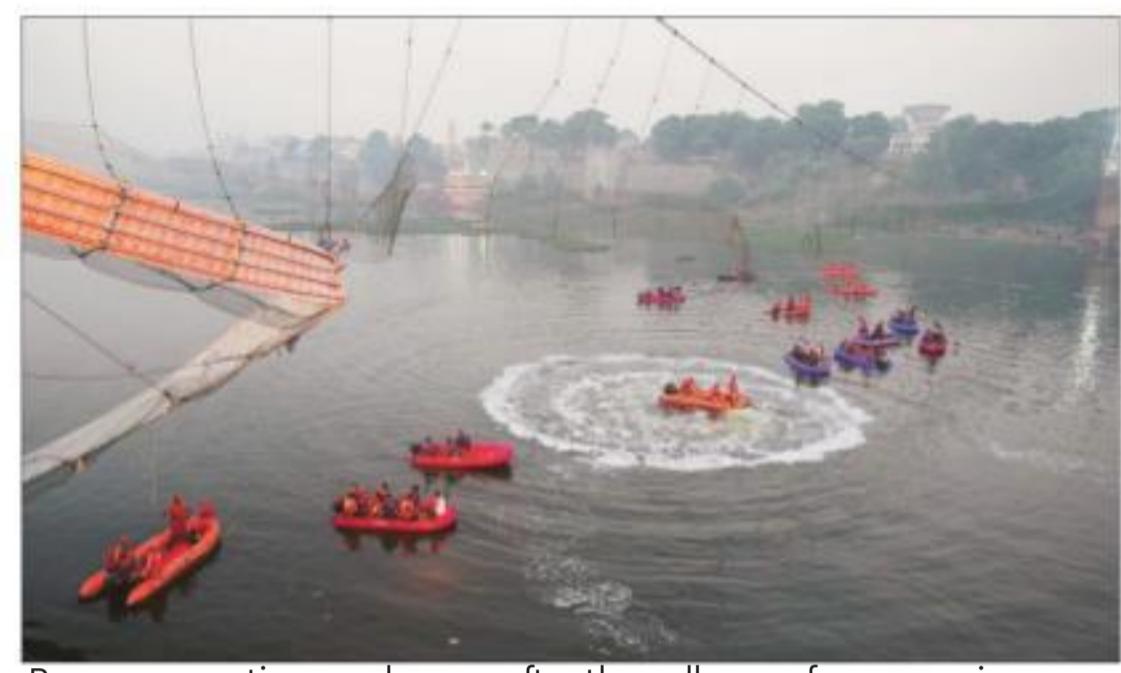
Rescue operations under way after the collapse of a suspension bridge over the Machchhu river in Morbi, Gujarat, on Monday
